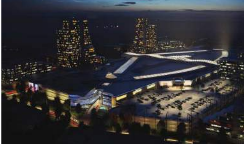
The 1.6mn square metre mixed-use Waterfall City, the most ambitious commercial development undertaken in southern Africa to date
