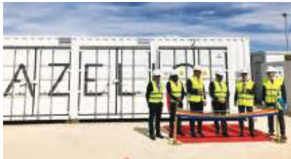
The renewable energy storage at the Noor Ouarzazate solar complex in Morocco.
