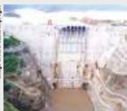
Ethiopia's Renaissance Dam will be the biggest in Africa.
