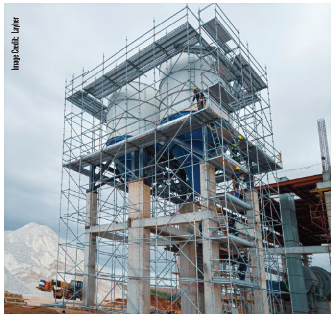
Layher Allround Scaffolding® assembled by MLS Scaffolding in Mozambique.
