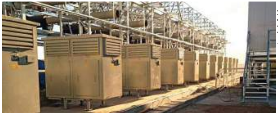
Transformers are housed in high protection enclosures, rated to IP44 or NEMA 3R, in an oil and gas plant project.
